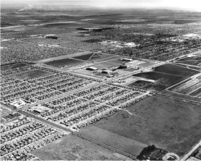
At the heart of Lakewood was a new shopping center (shown under construction in 1951). Its builders feared its annexation to Long Beach.
