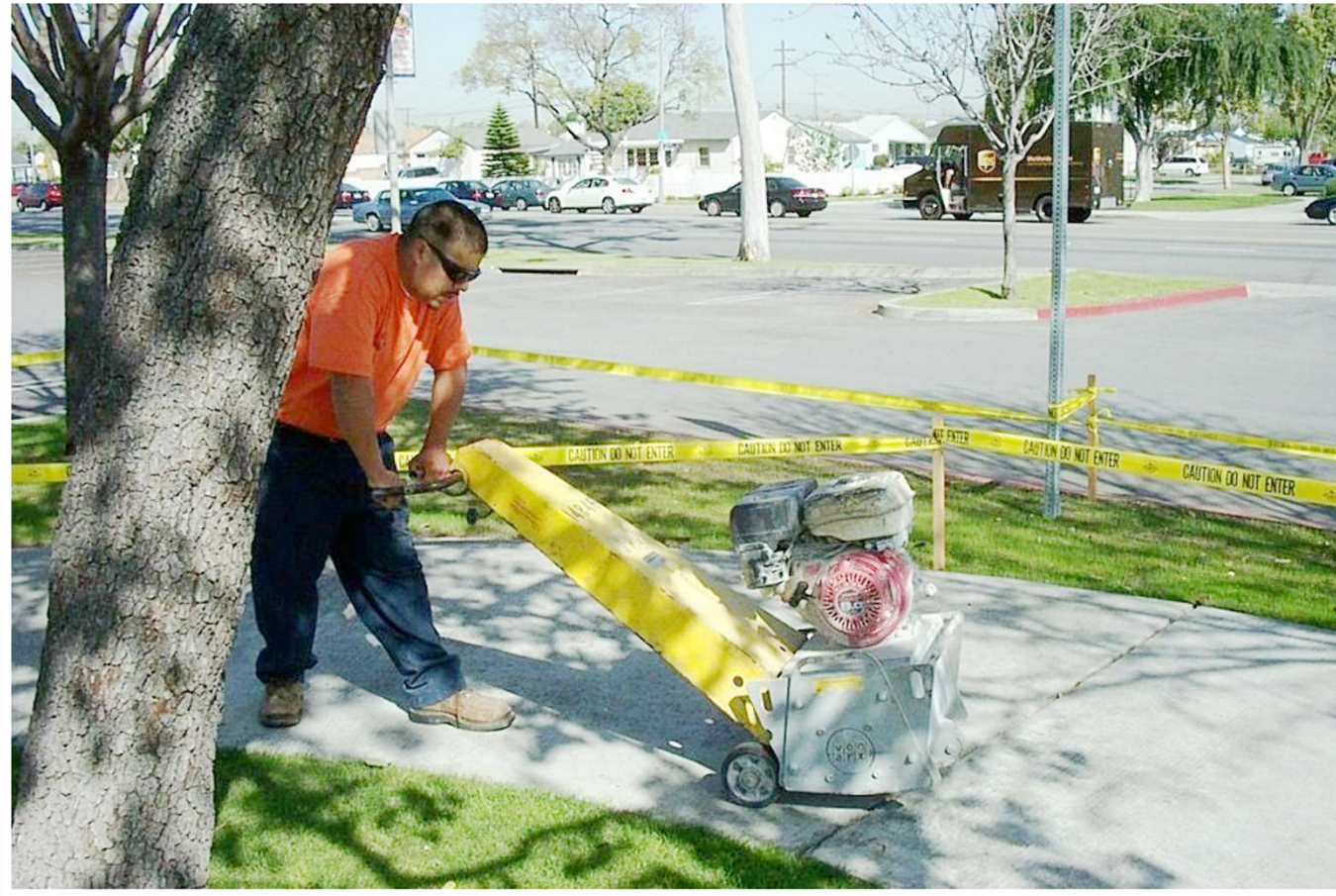
Sidewalk Grinding
